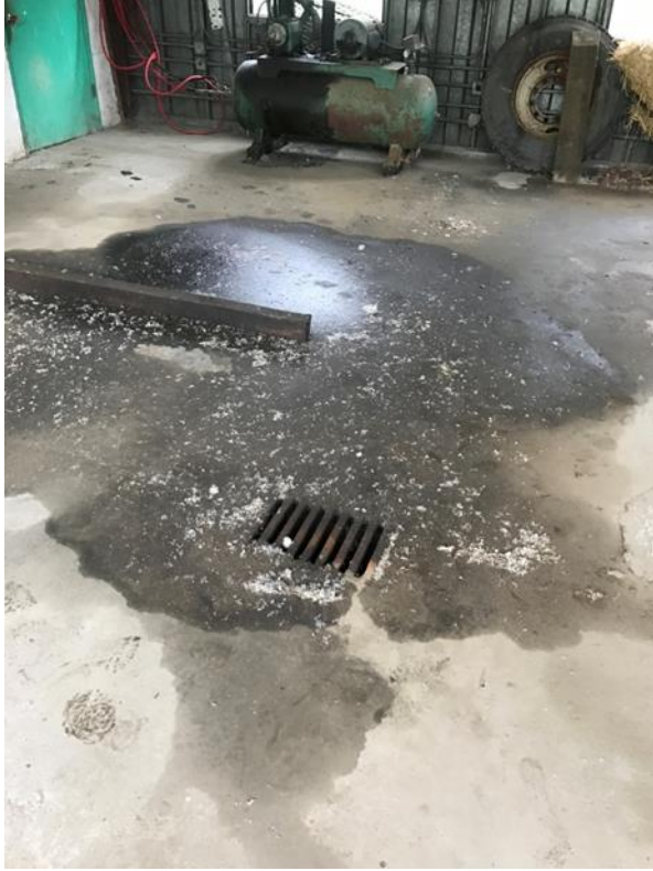
Figure 8. CB6 located in the equipment shop.
