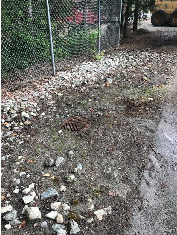
Figure 4. CB4, known as the washout station
