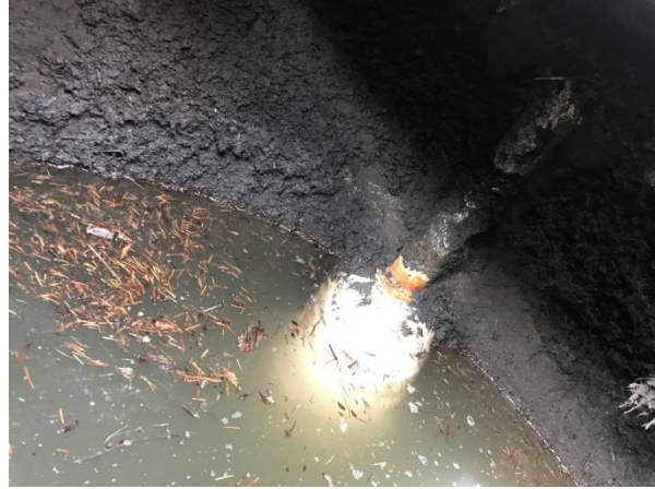
Figure 5. Possible oil-water separator within CB4.
