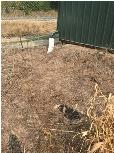
Figure 10. CB7 and one of two roof drains connected to CB7.
